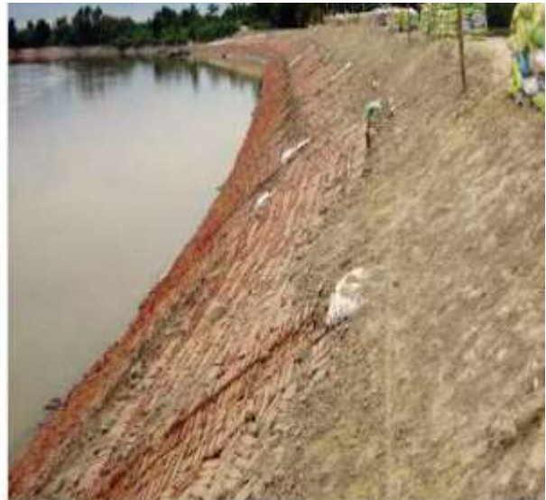
Raising & strengthening of Embankment on River, Burhi Gandak
