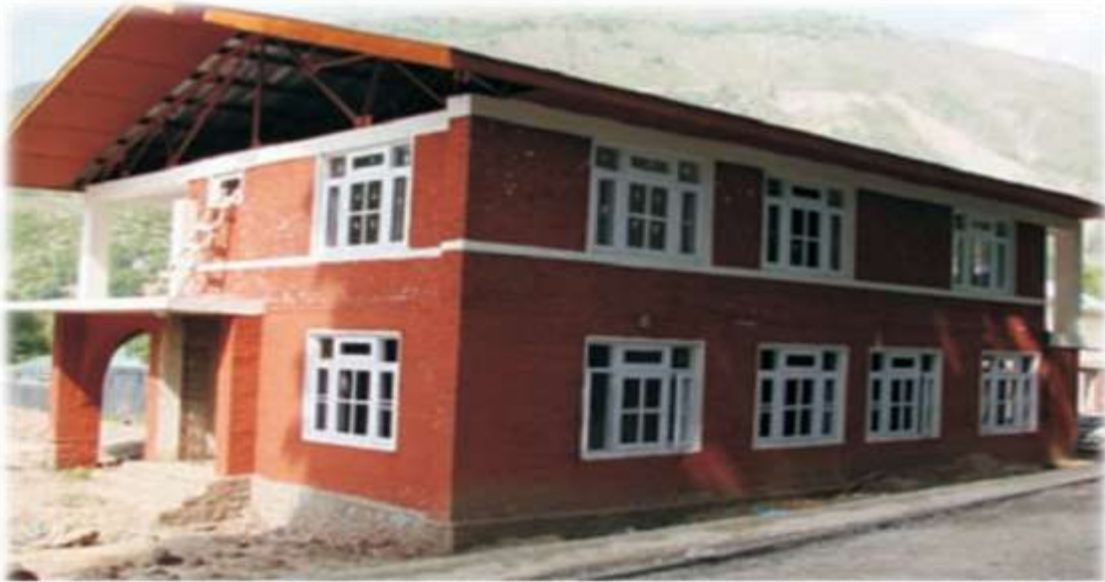
Jammu & Kashmir Earthquake 2005- Retrofitting on walls and windows
